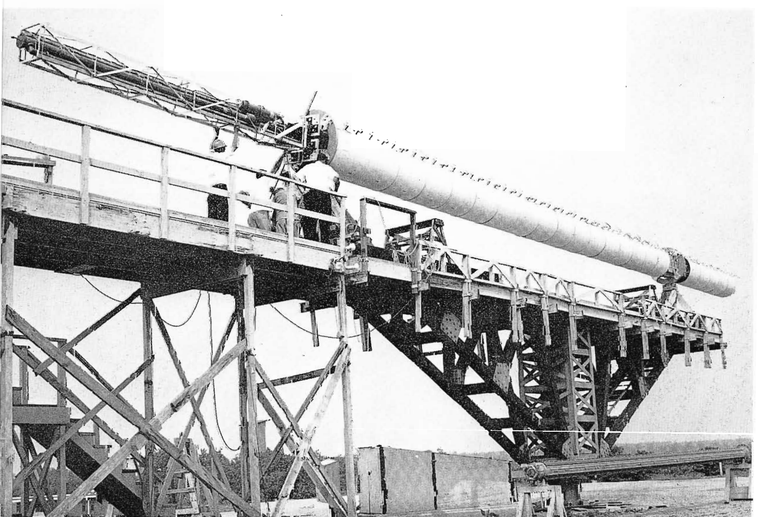
FIG. 6. WAND-TV antenna being pattern tested on turntable. Note antenna feed line assembly (seen at left in photo) located at the base of the antenna.
